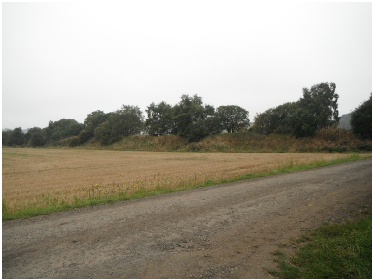
Photograph 9: Raised embankment at New Cottoun, east of Auchtertool.
