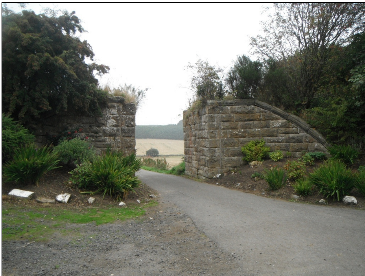
Photograph 7: Remains of abutments at track in the east of Auchtertool.
