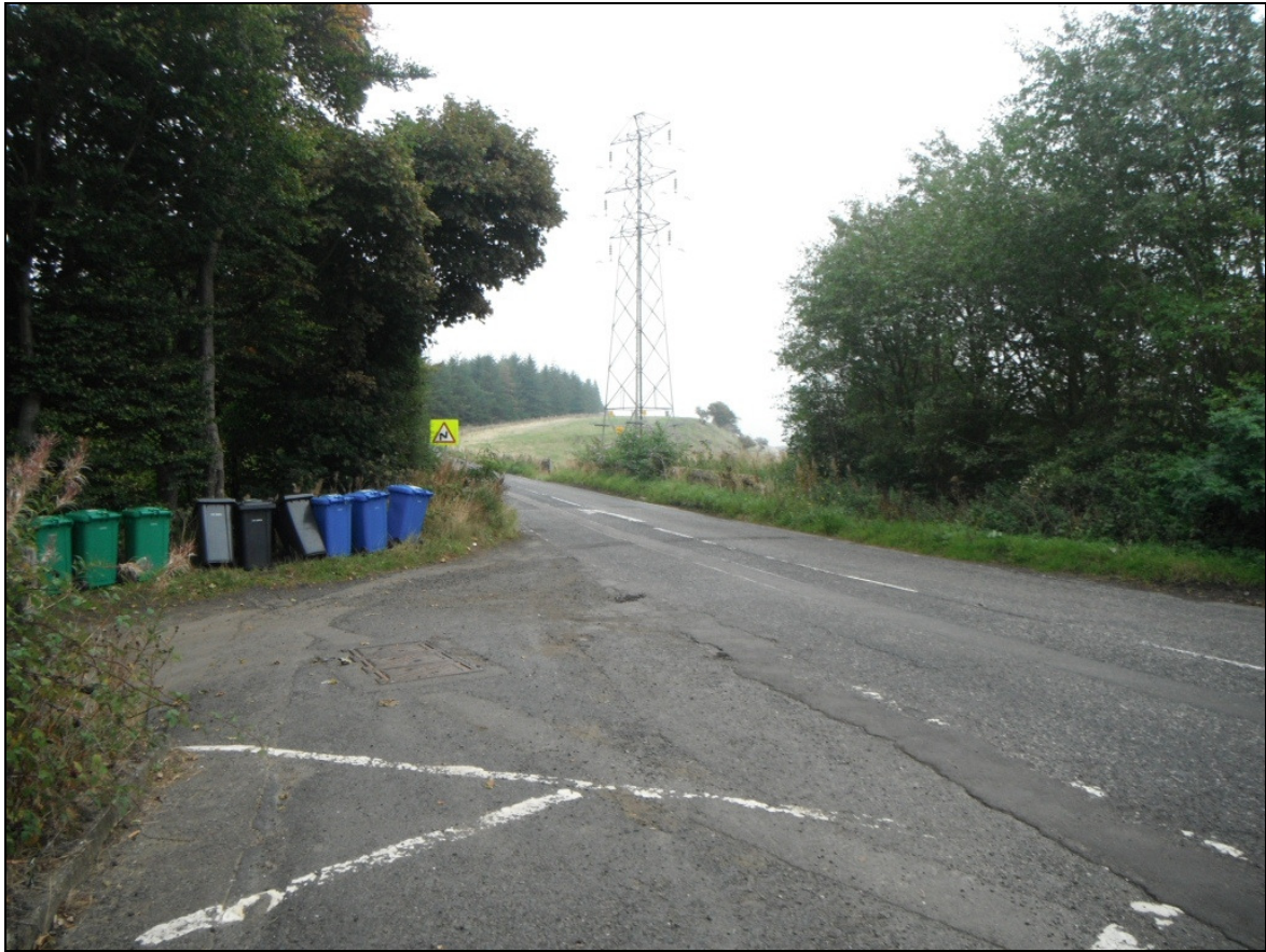
Photograph 11: Approximately location of where the former line crosses from the north of the road (B 825 at Balbarton) to the south.
