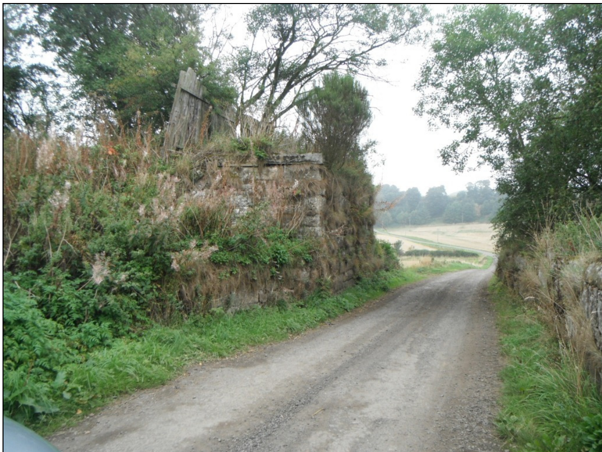
Photograph 10: Remains of abutments at New Cottoun.
