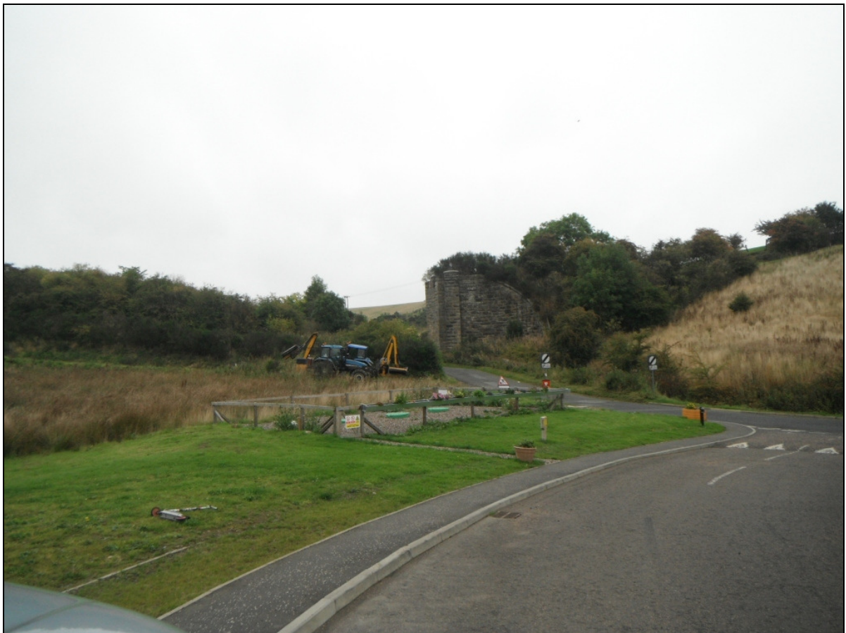
Photograph 5: Remains of abutment where raised rail line would cross above the road.
