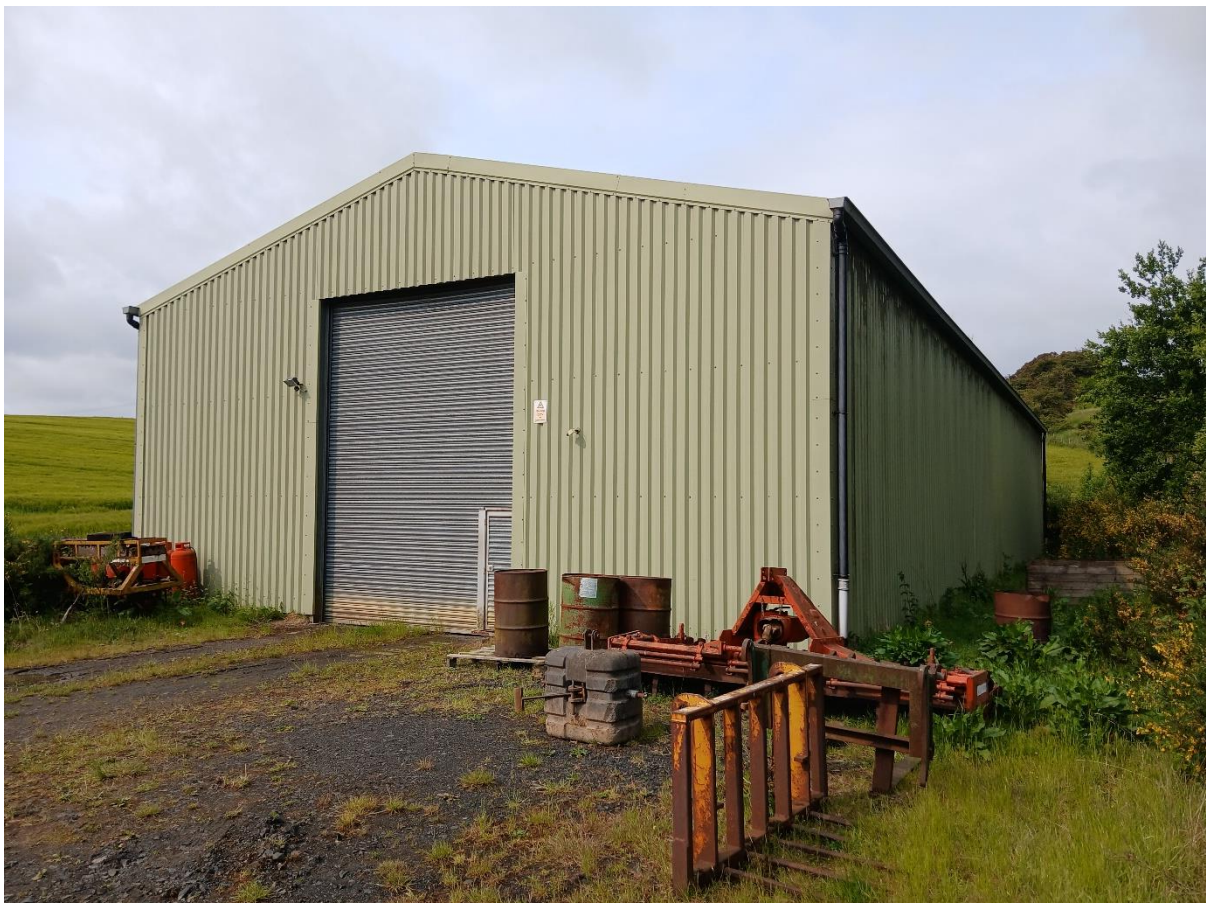
Plate 2: Photo looking at Metal barn associated with Camilla Farm in the southeast of site.
