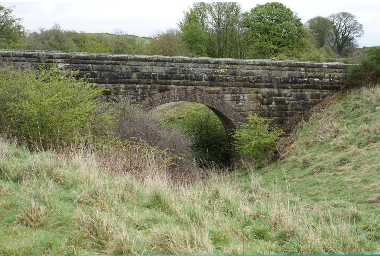
Figure 6.8 Stone bridge with brick archway
