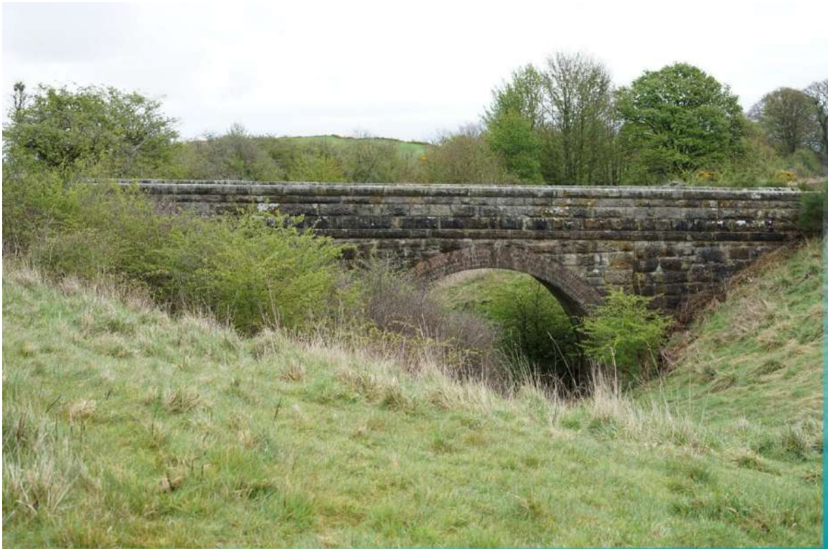
VP10 Railway bridge looking east, illustrating drop in land levels
