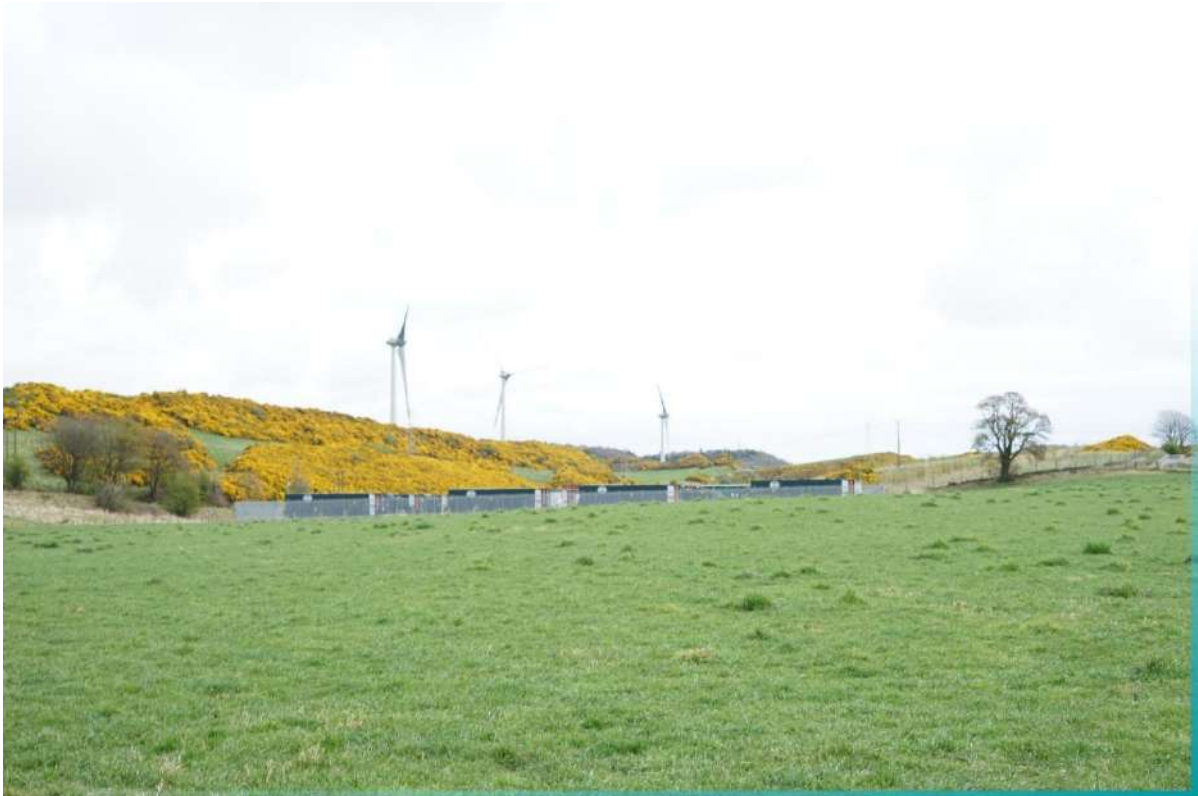
VP13 Photo looking northeast, toward Camilla BESS and windfarm beyond
