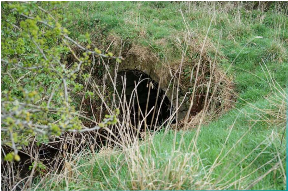
VP8 Photo showing stone bridge at edge of agricultural field - not accessible due to fencing
