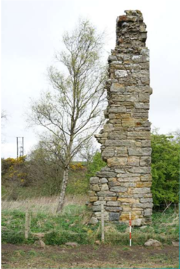
VP12 Approximately 7m high section of wall remaining upright at Camilla: Castle
