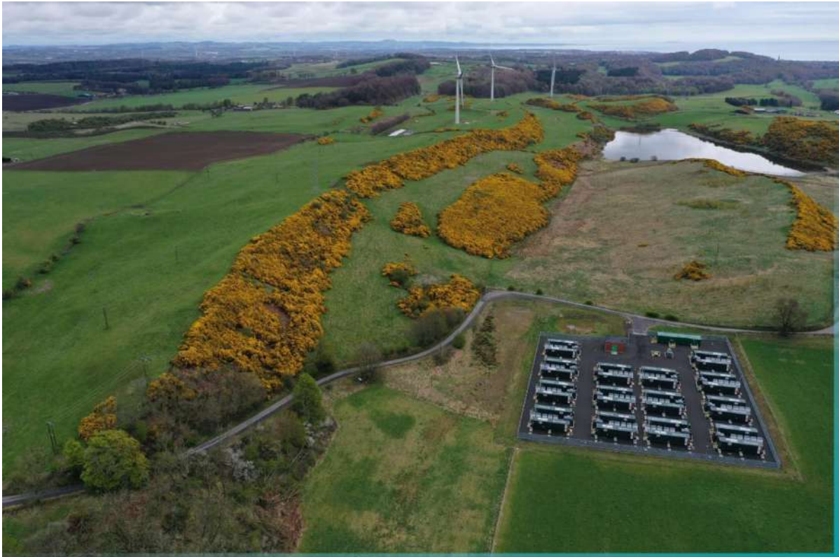
VP19 Drone photo of Camilla BESS site
