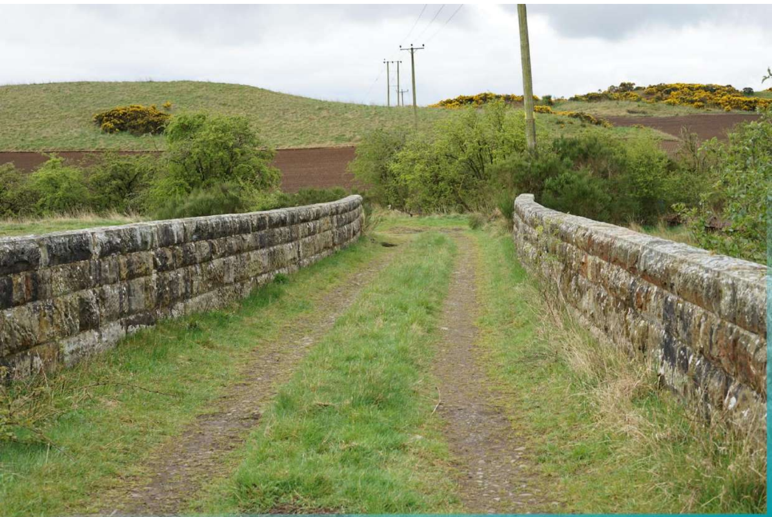
Figure 6.7 Bridge over dismantled railway
