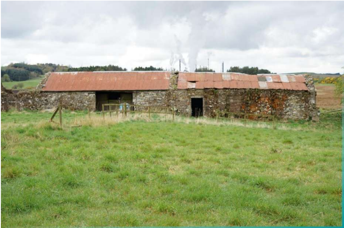
VP17c Camilla: Building, middle section which appears in occasional use to house livestock
