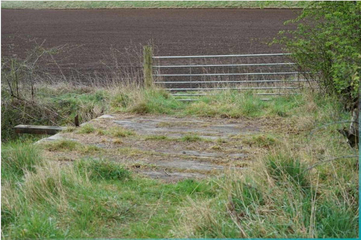
VP9 Wooden footbridge, appears to be constructed of repurposed railway sleepers
