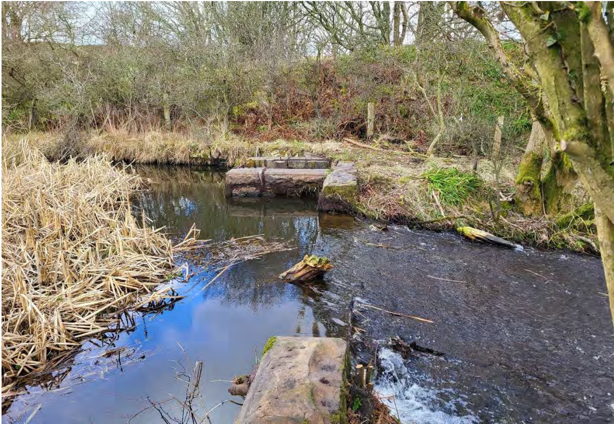
Photo 9: Weir on Dronachy Burn
