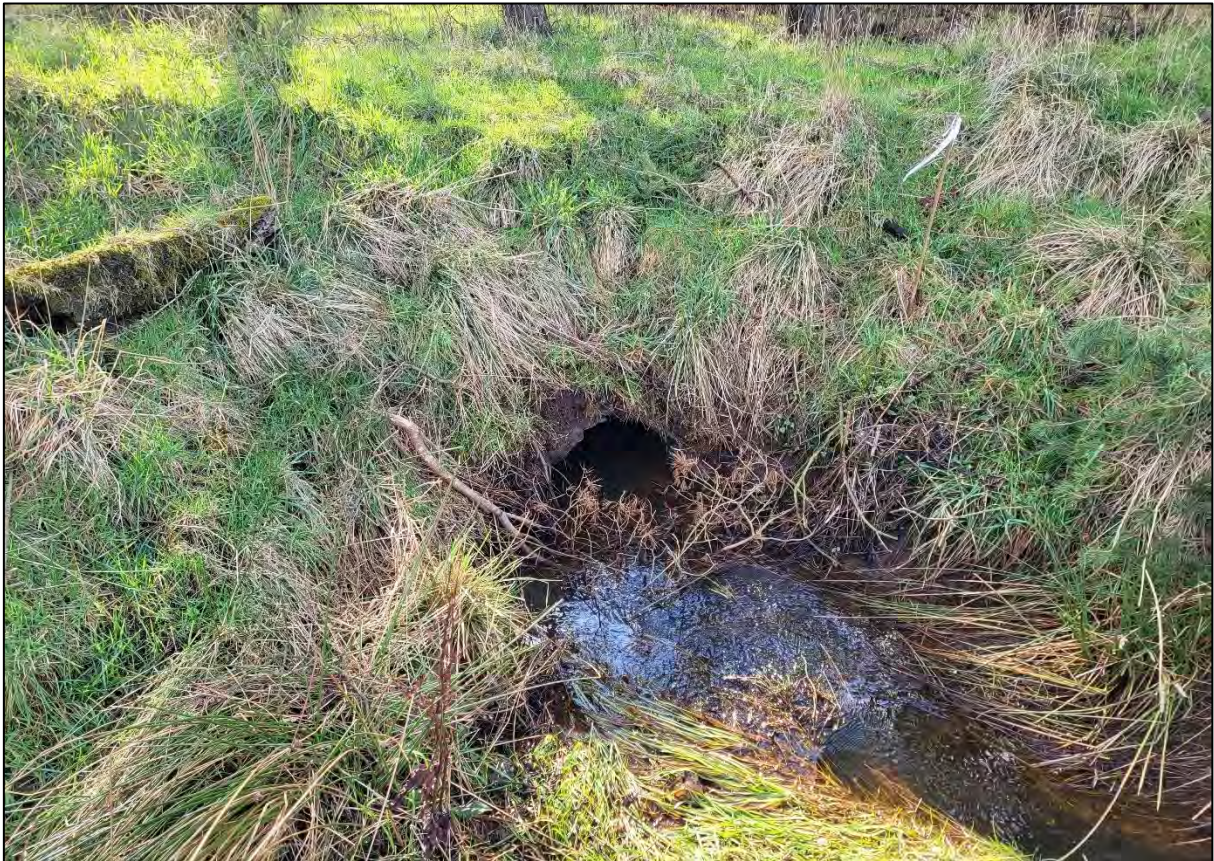
Photo 5: 0.62m Diameter Culvert under former railway embankment
